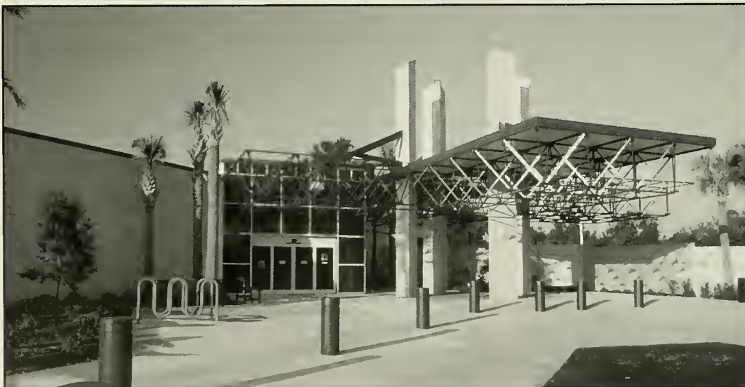
A brightly colored space frame identifies the front entry. Shadows play across the partly covered/partially open sidewalk. Photograph: Bruce Gora
